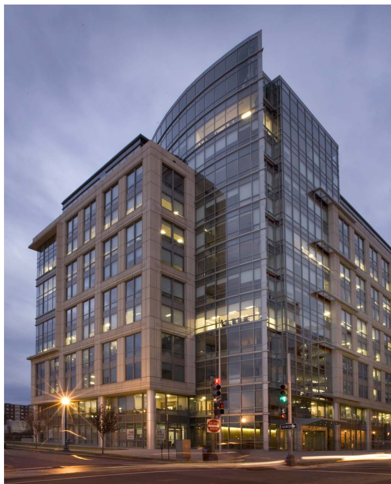
Capital Plaza, Washington D.C. LEED® Rating: Platinum
