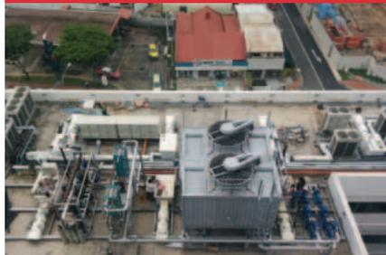
**Air Conditioning System Retrofitting** – Conversion of air cooled VRV system to centralised water cooled refrigeration system to achieve efficiency of 0.67 kW/RT with estimated reduction of energy consumption at 848,985 kWh/year (about 33% reduction).
