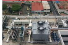
Air Conditioning System Retrofitting – Conversion of air cooled VRV system to centralised water cooled refrigeration system to achieve efficiency of 0.67 kW/RT with estimated reduction of energy consumption at 848,985 kWh/year (about 33% reduction).
