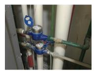
Each unit has 2 water meters, 1 meter for municipal water consumption, another for grey water consumption.
